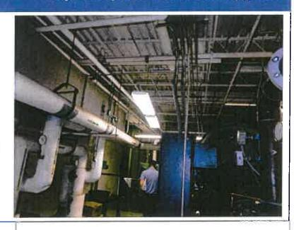
The 30-plus year old chiller serving Building 36 failed in the spring of 2016. MEI was retained to design the installation of a temporary rental chiller, which remains in service at this time. MEI was then retained to design a full HVAC retrofit to the building due to the condition of the
